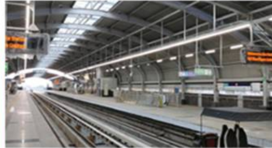
Kolkata Metro Project, West Bengal, India
