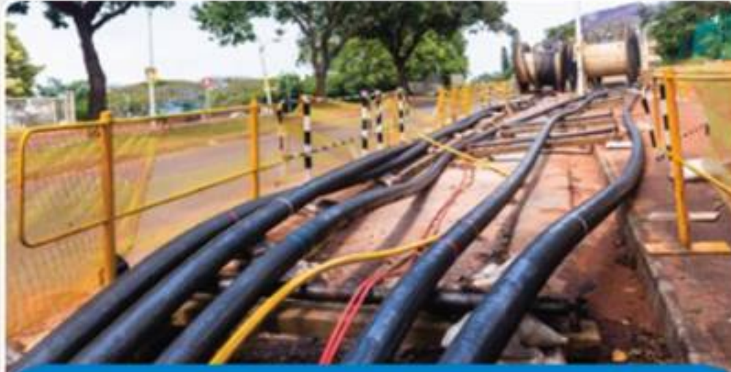
Underground Cabling Works in Rampur, Uttar Pradesh, India
