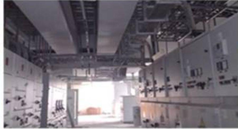
Bengaluru Metro Project, Karnataka, India
