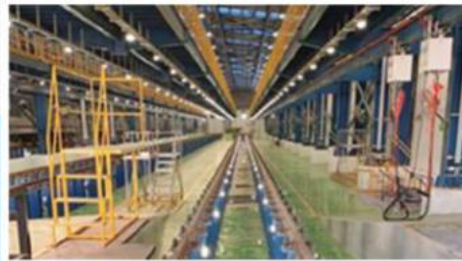
Mumbai Metro Project, Maharashtra, India
