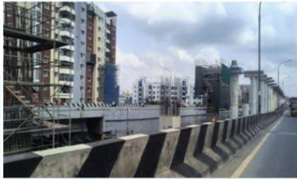
Chennai Metro Project, Tamil Nadu , India
