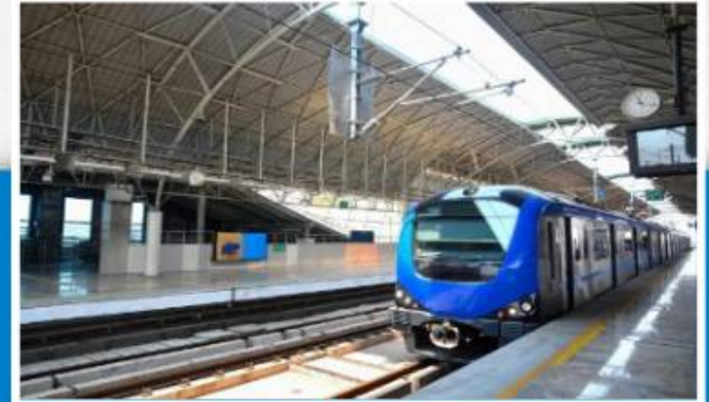
Chennai Metro Project, Tamil Nadu , India
