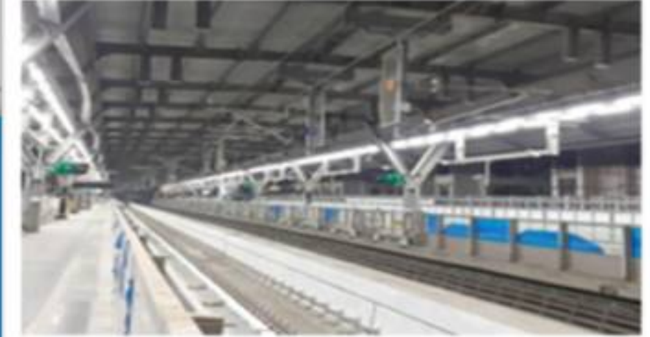
Mumbai Metro Project, Maharashtra, India
