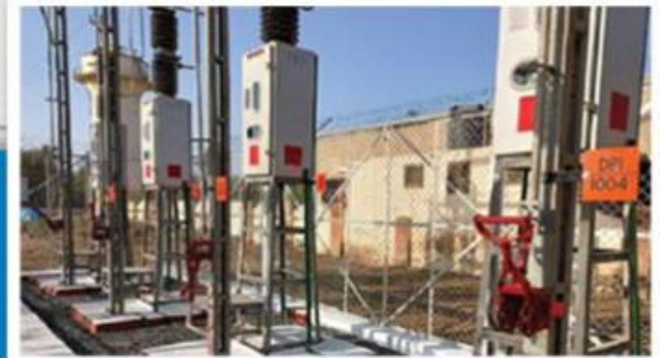
Overhead Railway Electrification under CORE Project
