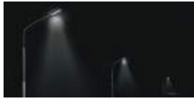
STREET LIGHT INSTALLATIONS UNDER SLNP*
