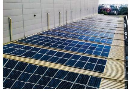
the 2010 Commonwealth Games. YSC wanted to harvest the power of solar. However, the metal roofing of the complex posed a challenge for installing solar panels. This was overcome by Jakson using innovative engineering capabilities. The plant consists of 1600 modules of 250 Wp capacity which generates approximately 5.84 lakh units per year. Bi-directional meters are installed for sale of power to the grid in case of surplus.
