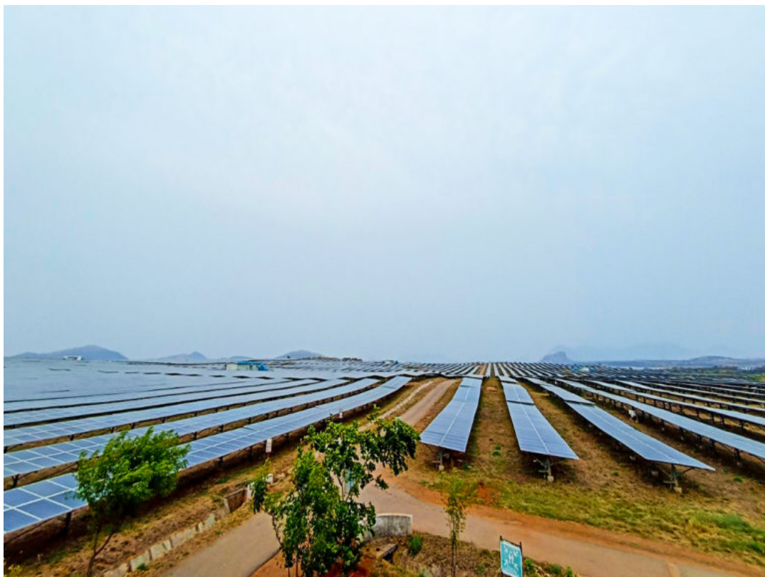
NTPC's 250 MW Ananthapuram solar project
