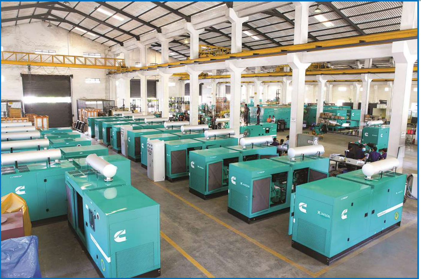
A Genset manufacturing Unit of the Jakson Group
